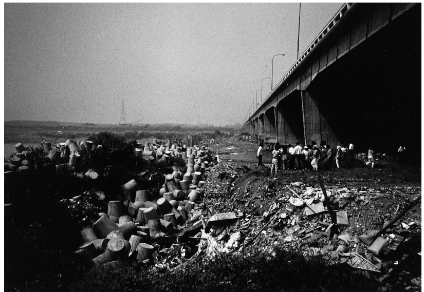
Figure 13. Undercutting and grade control efforts along the downstream side of the Kaoping Bridge over the Kaoping River, Taiwan, to control incision caused by massive gravel mining downstream. (Photograph by the author, October 1995.)
