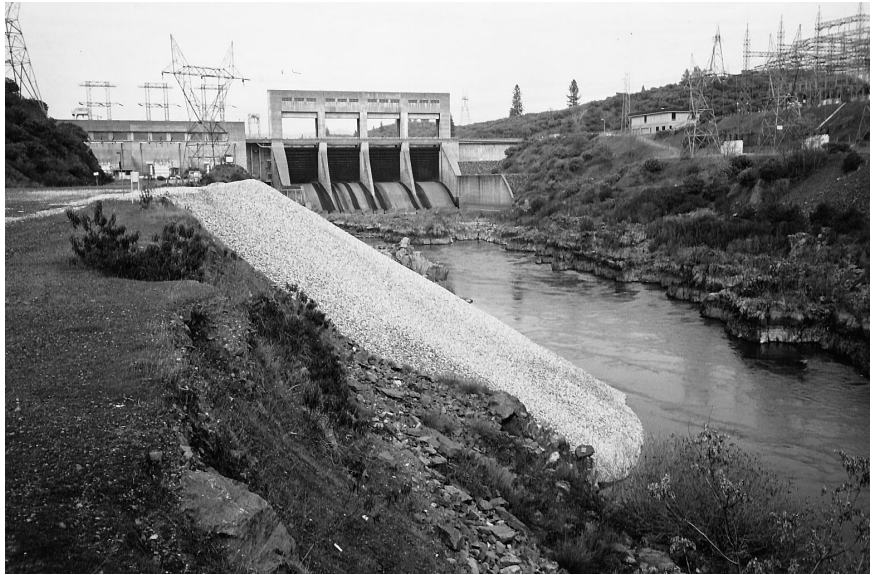
Figure 4. Gravel replenishment to the Sacramento River below Keswick Dam. (Photograph by the author, January 1991.)
